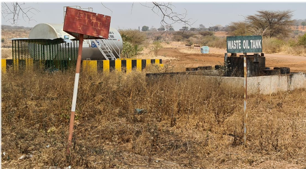
Figure 10: Used Oil Receiving Tank
